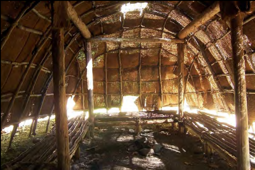
Native American Long House (restored)
