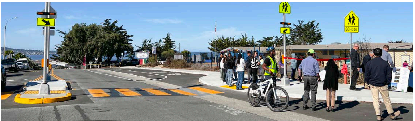
Pedestrian improvements at the Ord Terrace Elementary School were implemented in 2023.
