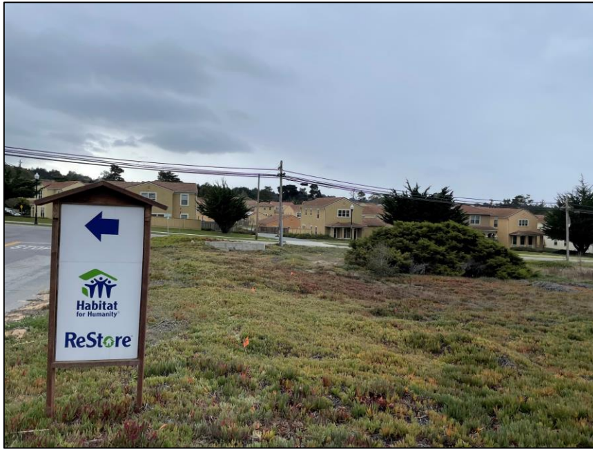
Photo 5: Eastern edge of property, looking south.
