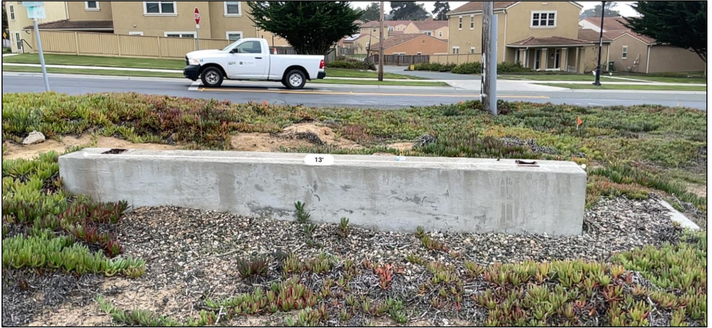
Photo 7: View of concrete berm, looking south.
