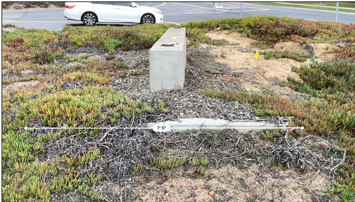
Photo 8: View of concrete pad, looking west.
