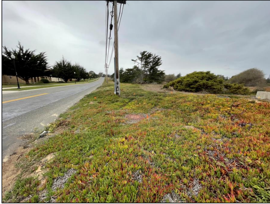
Photo 9: View of orange flags and manhole for AT&T underground communication lines.
