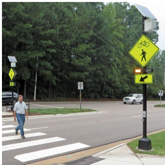
Safety Enhanced Crosswalks
